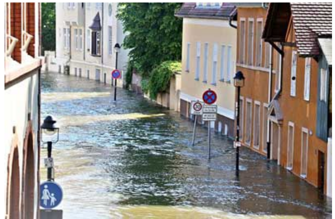
A flooded street in Halle, spring 2013
